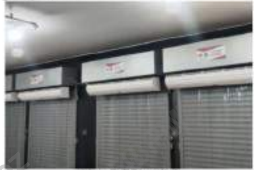
Air curtains installed
